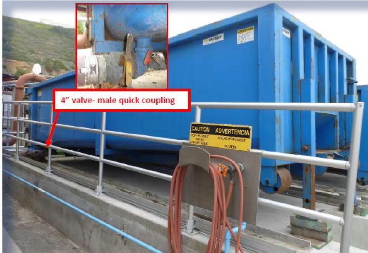
The containers at NCWRP shall not exceed 19 feet in length and not exceed 7 feet in height. The North City wet sewage scum container fill hatch shall be on the left rear (drivers) side and top of the container which will accommodate the NCWRP fill line to fill the container. The container shall have a bottom decant line with a valve on the bottom of the container used for decanting as described above. See attachment photo for example.
