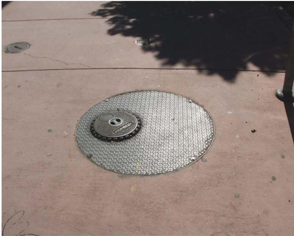
1) View of diesel underground storage tank fill port in sidewalk (Building A).
