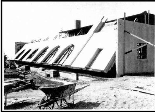
The La Jolla Women's Club was designed in 1913 by Master Architect Irving Gill, and is a significant example of Gill's interest in building technology. The building was constructed using a tilt-slab reinforced concrete wall system, which allowed entire walls containing doors and window frames to be tilted into place and then finished
