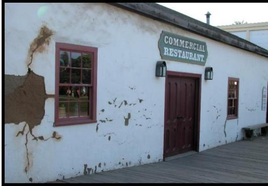
The Casa de Machado is an adobe house built in 1832 by Jose Manuel Machado as a wedding present for his daughter. The foundation is constructed of field stone laid in adobe mortar. The walls consist of sun dried adobe brick laid in adobe mortar, plastered on both sides with adobe mortar and white washed.
