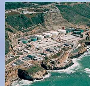
Point Loma Wastewater Treatment Plant
