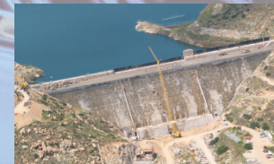
San Vicente Dam Raise Construction
