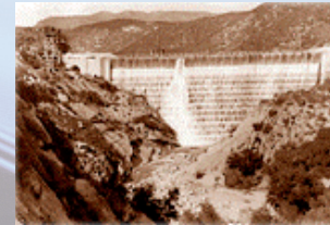
Barrett Dam (built in 1922)
