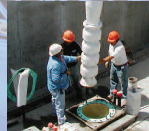
Groundwater Well Installation
