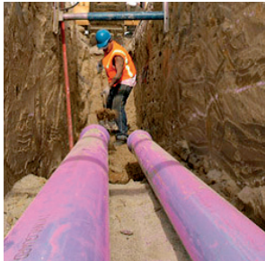
Installing purple pipes for non-potable reuse
