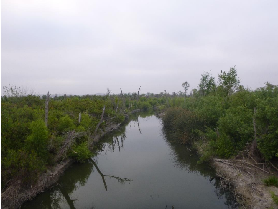
9. Looking upstream in Pilot Channel from the Hollister Street Bridge. Some debris was seen at the bridge abutments.
