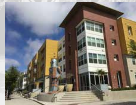
Increasing Access to Affordable Housing
