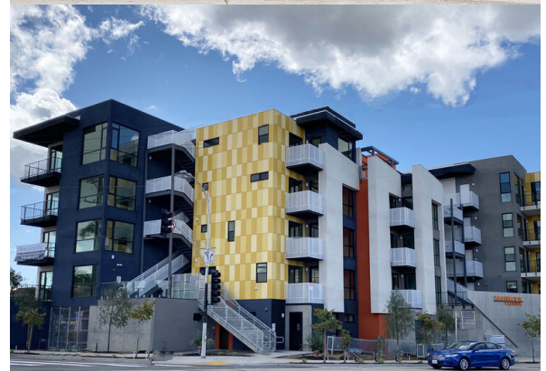
Washington Crossing in Uptown was permitted in 2018 for the development of 36 units, three of which are dedicated as affordable to veterans and foster youth. The photos shown are of the project construction, taken in 2019 and the completed project, taken in 2020.
