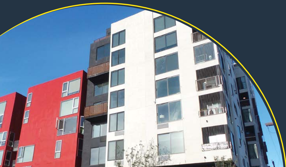
Harvey Apartments, located in Hilcrest.
