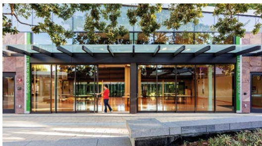
An example of a retractable door connecting a community room to an outdoor terrace.
