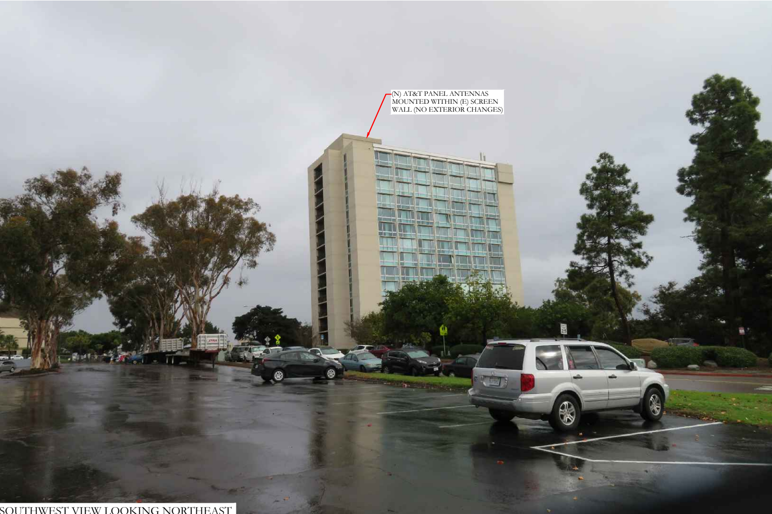
SOUTHWEST VIEW LOOKING NORTHEAST
