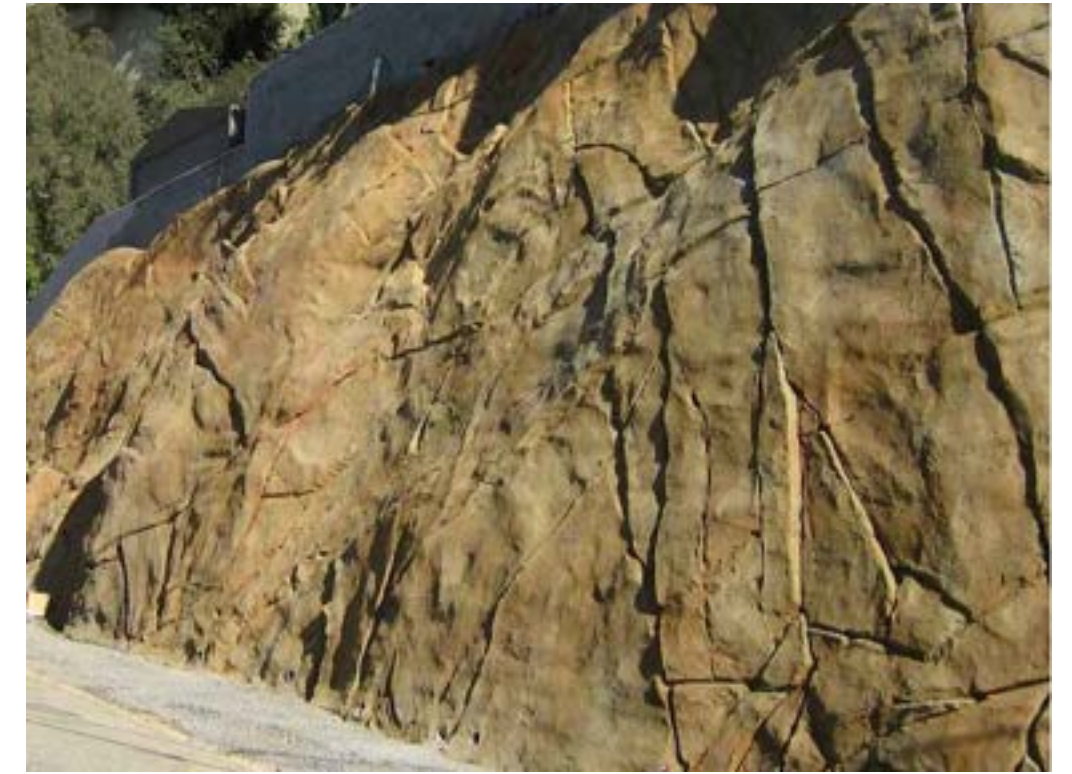
RETAINING WALL ALONG ENTRY ROAD (CUT SLOPE) SITE WALLS
