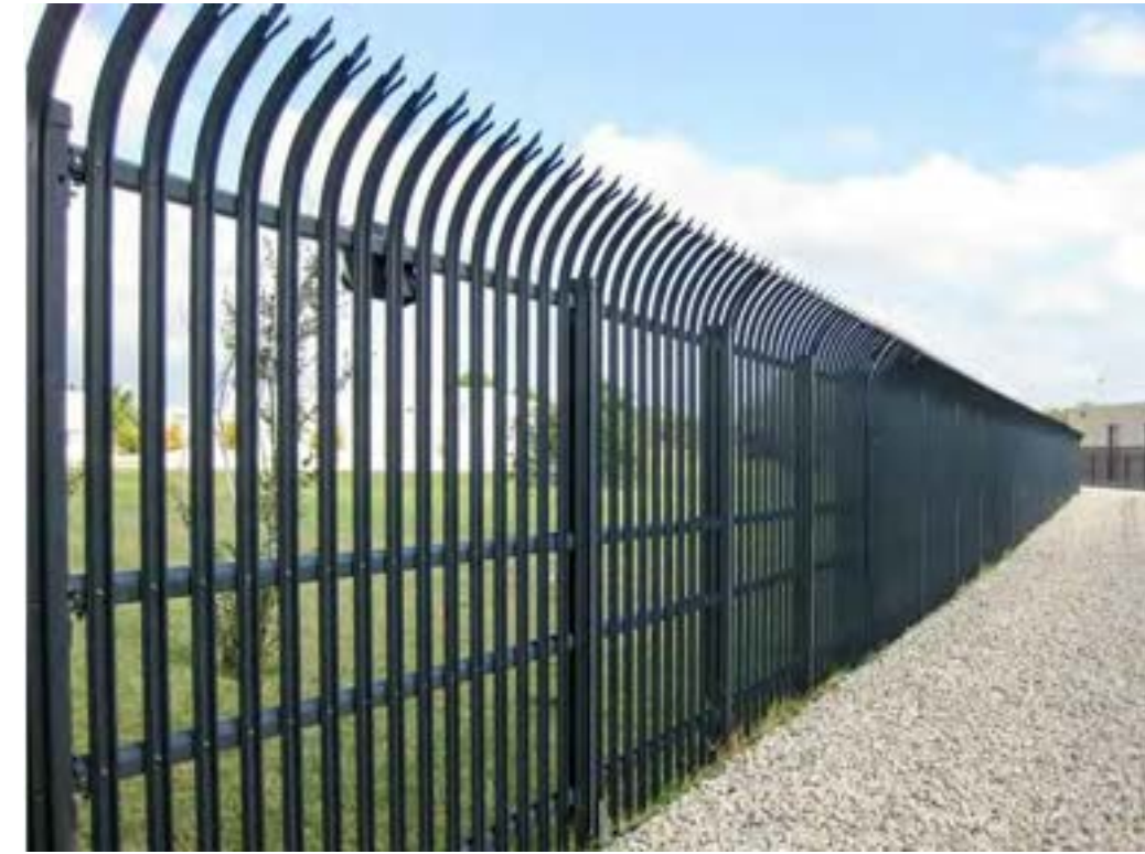
SECURITY FENCING AT SDCWA VENTS FENCING
