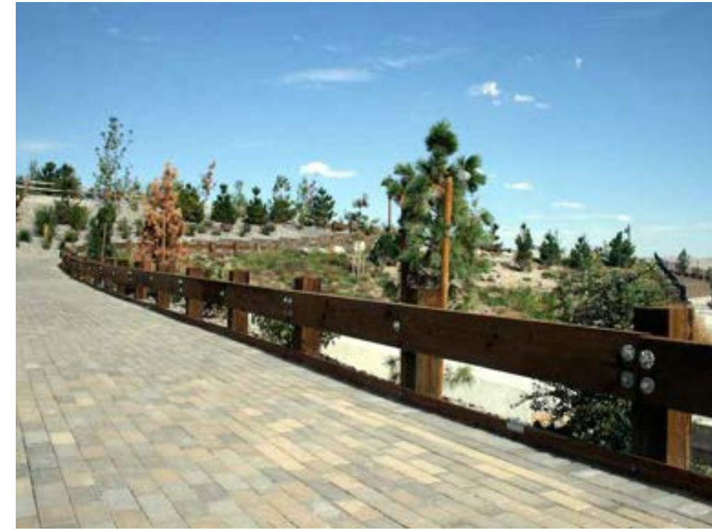
GUARDRAIL ALONG ENTRY ROAD GUARDRAIL
