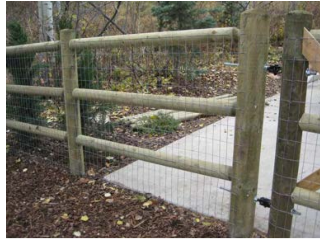
LODGE POLE PINE FENCING WITH CHAINLINK MESH FENCING
