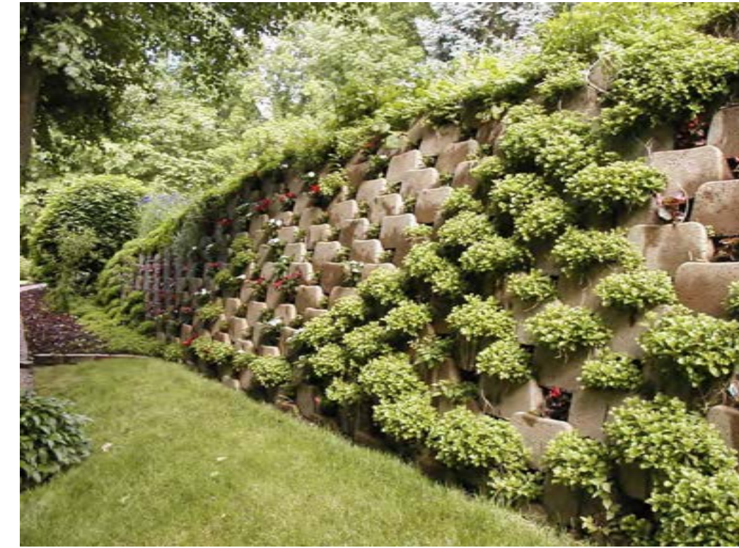
RETAINING WALL ALONG ENTRY ROAD (FILL SLOPE) SITE WALLS
