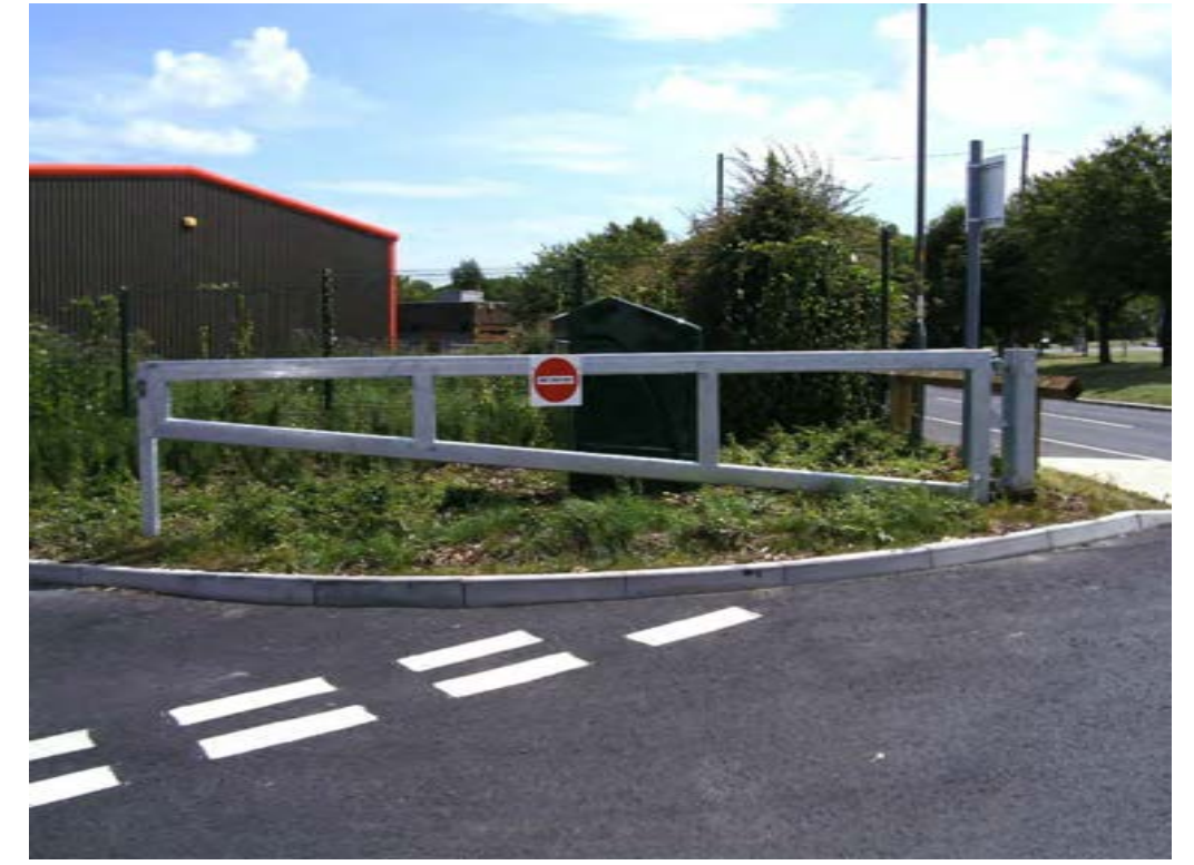
SWING GATES AT SERVICE ROAD TRAILS GATES
