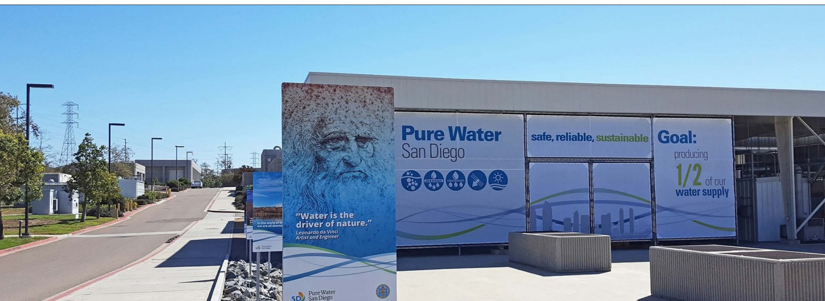
The Pure Water Demonstration Facility
