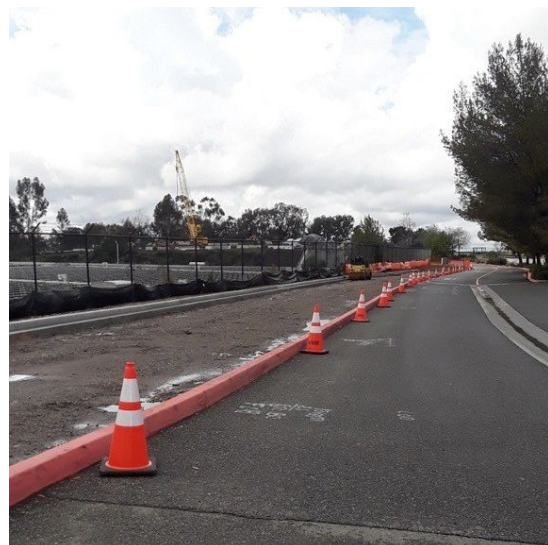
Restoration underway at the Miramar Reservoir parking
