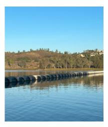
Did you know? The Subaqueous Pipeline is 4.5 feet in diameter with smaller pipe "branches" that will be installed to ensure that the purified water is equally dispersed throughout Miramar Reservoir.
