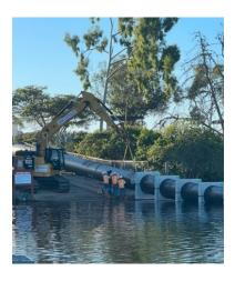
Construction crews fuse pieces of pipe together on land and string it out on Miramar Reservoir before installing it on the lakebed.
