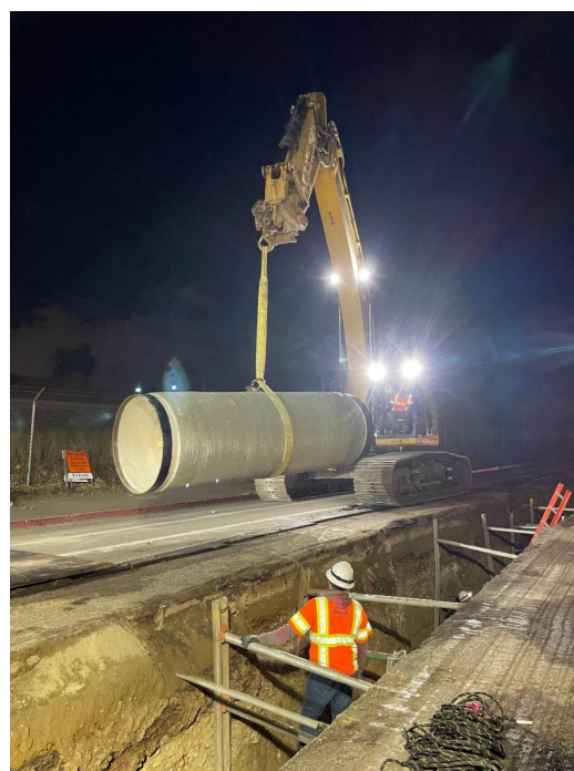
Nighttime pipeline installation on Miramar Road.
