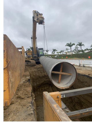
Pipeline construction on Clairemont Drive.
