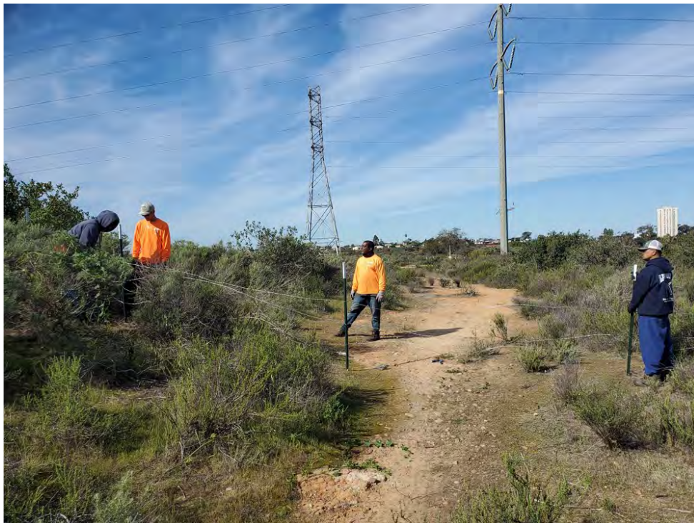
Photo 67. Contracted crew performing fence installation.
