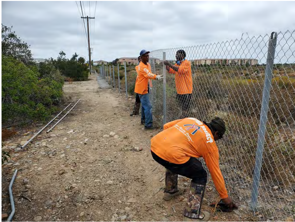
Photo 6. Contracted crew performing fence repair.
