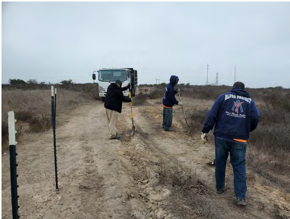
Photo 70. Contracted crew performing fence installation.
