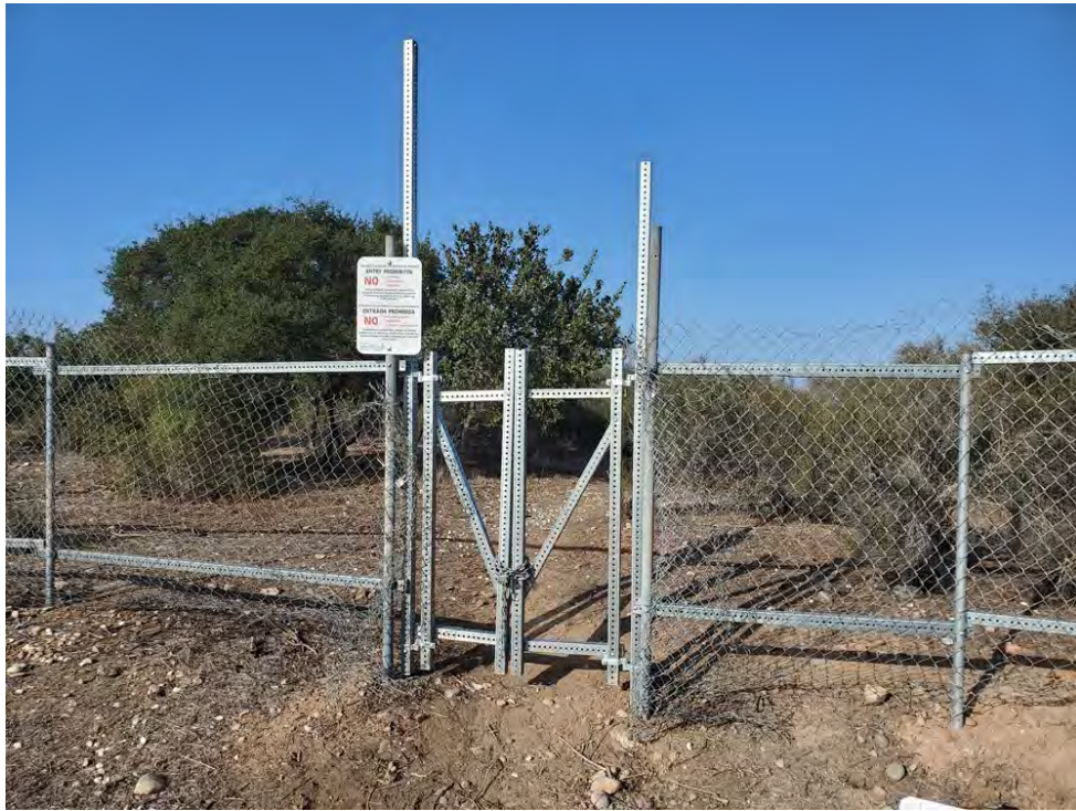
Photo 26. City staff performing gate installation.
