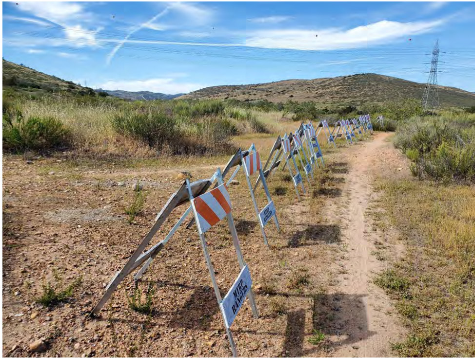
Photo 64. City staff installed barricades to block access into vernal pools.
