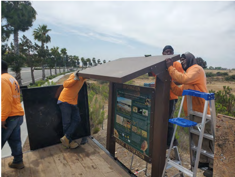
Photo 20. Contracted crew performing kiosk installation.
