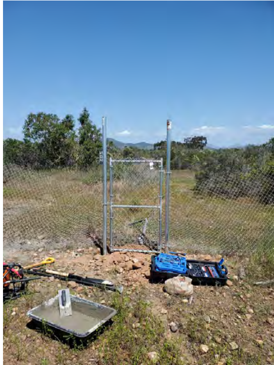
Photo 25. City staff performing gate installation.
