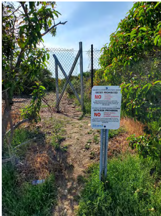
Photo 53. City staff performed sign replacement and fence repair.
