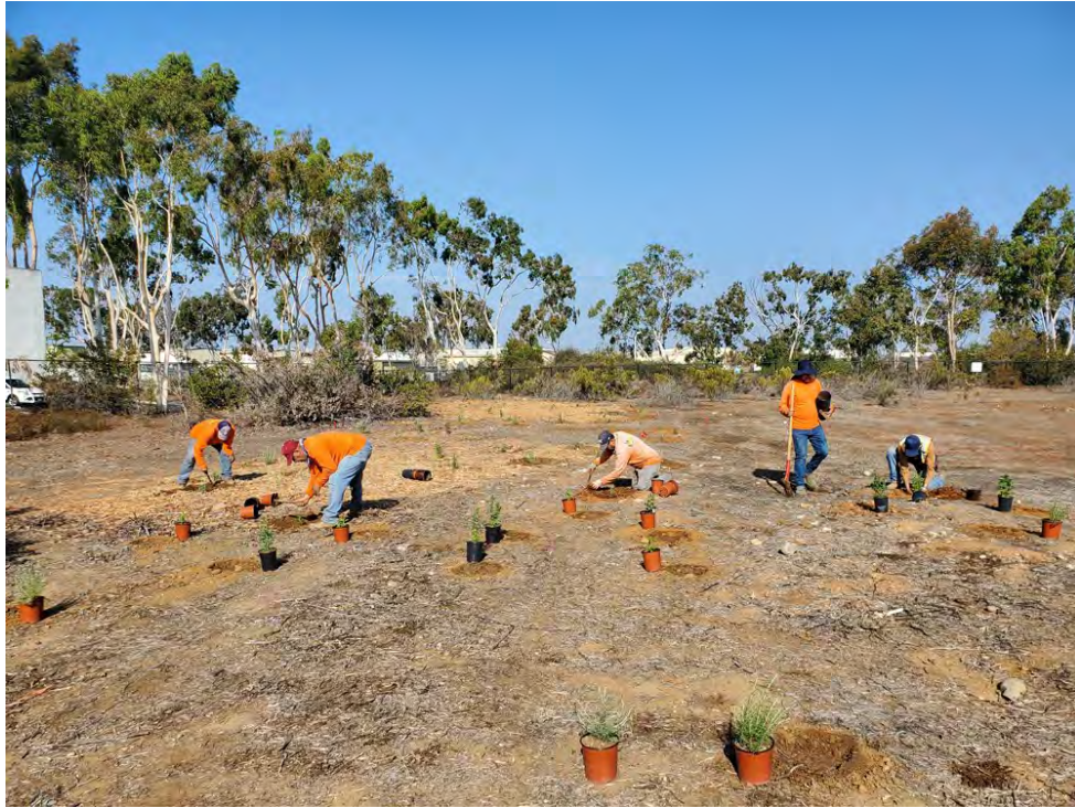
Photo 60. Contracted crew performing plant installation.
