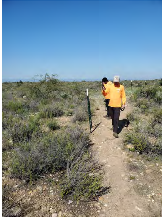
Photo 57. Contracted crew performing fence installation.
