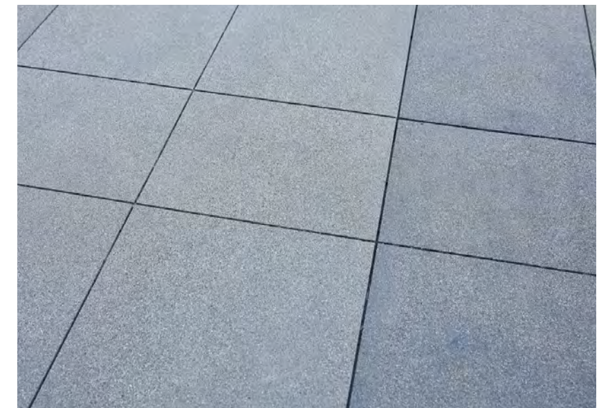
E Street Paving
