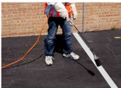
*proposed material- road marking strips for temporary installation of 2-5 yrs
