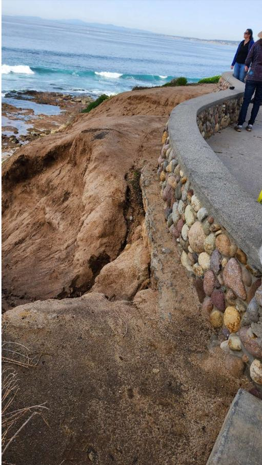
Looking north towards wall footing and slope erosion
