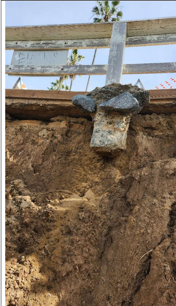
The rail footing exposed, with sidewalk undermining looking up slope.
