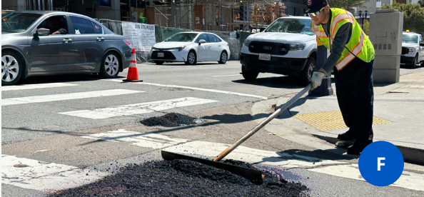
Figure 1-3. Pavement Repair Method Examples: A) Crack Seal B) Slurry Seal; C) Cape Seal; D) Scrub Seal; E) Mill and Pave; F) Pothole Repair
