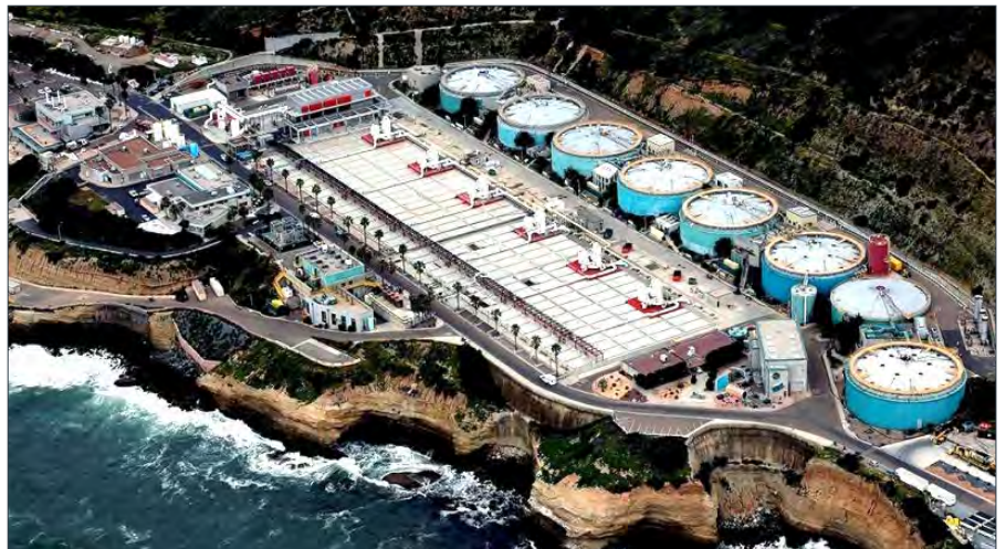
The Point Loma Wastewater Treatment Plant
