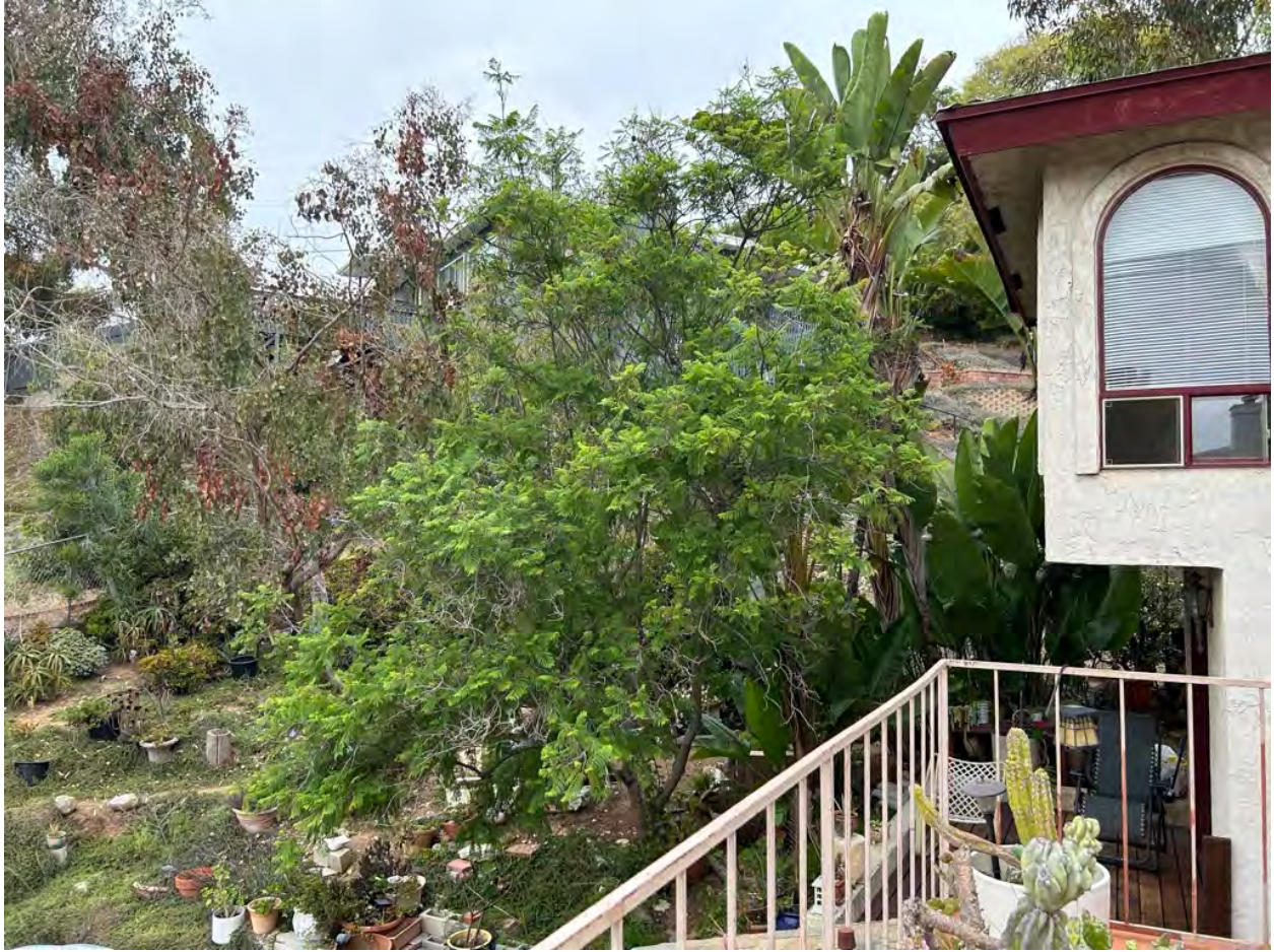
Foreground is Sharon's Lanai and bedroom window above. Behind it is the construction area.
