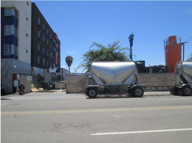
1. Southerly view of the Site entrance on Imperial Avenue.
