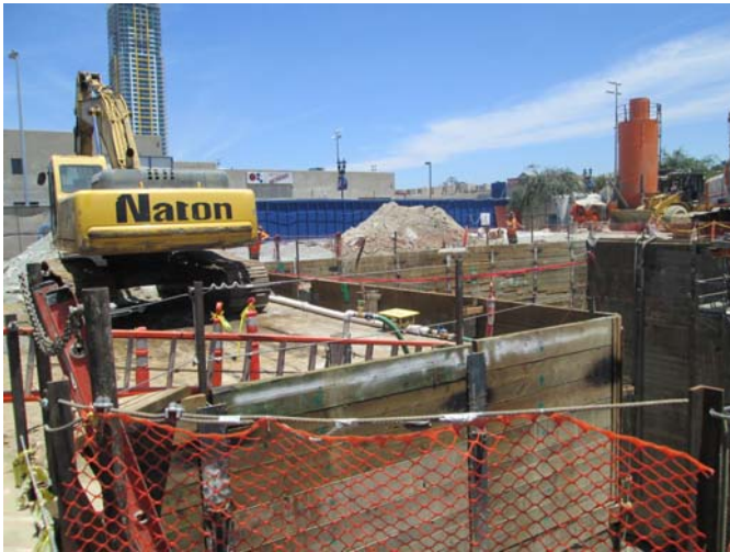
7. Excavation and construction equipment.
