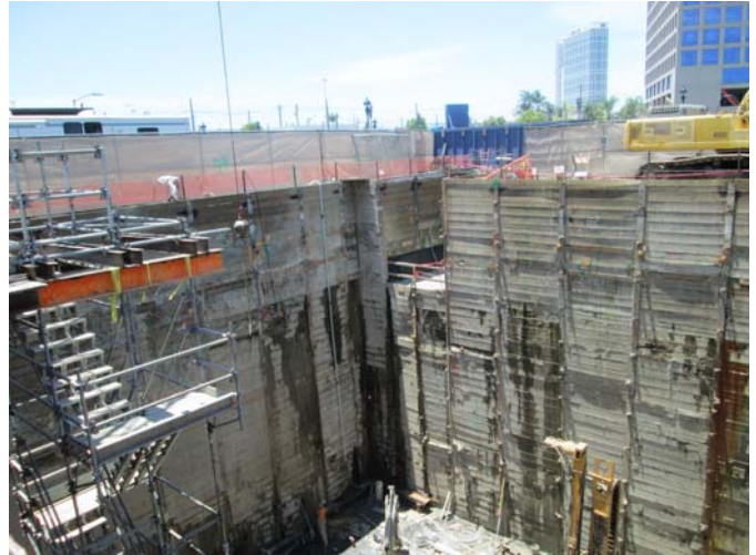
4. View of the shored excavation.
