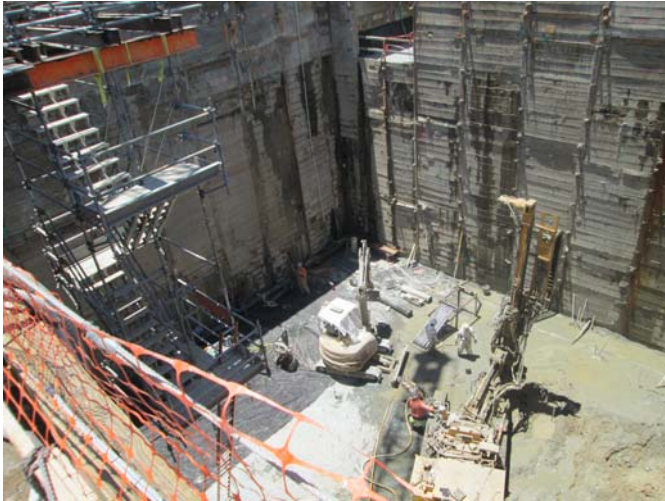
3. View of the shored excavation.
