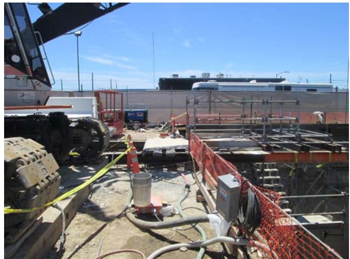
6. Excavation and construction equipment.
