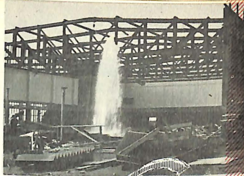
NOT "OLD FAITHFUL", JUST A BROKEN PIPE AT CALLAN
