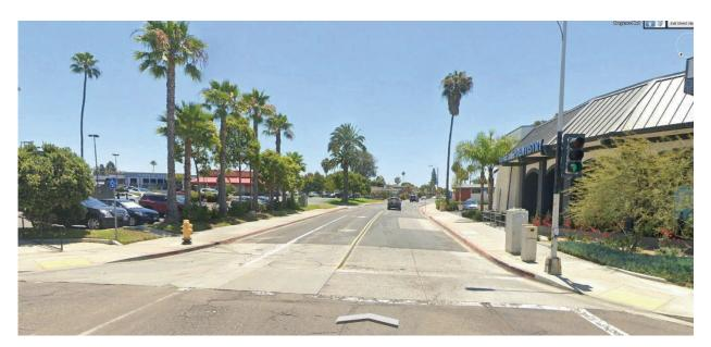
**Field Street** – Contiguous sidewalk exists on both north and south sides of the street segment between Burgener Blvd. and Cowley Way. Crosswalks are provided on all four legs of the all-way stop controlled intersection of Field Street / Burgener Boulevard. Single curb ramps with truncated domes exist on the northwest, northeast, southwest, and southeast corners of the intersection of Field Street / Burgener Boulevard.
