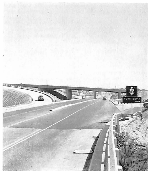
Mission Valley Road Overpass Completed during the year to provide fast movement of traffic.
