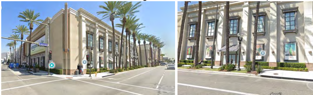
Colorado St. & Central Ave at Americana @ Brand w/ fake windows and doors for building articulation along the surrounding streets
