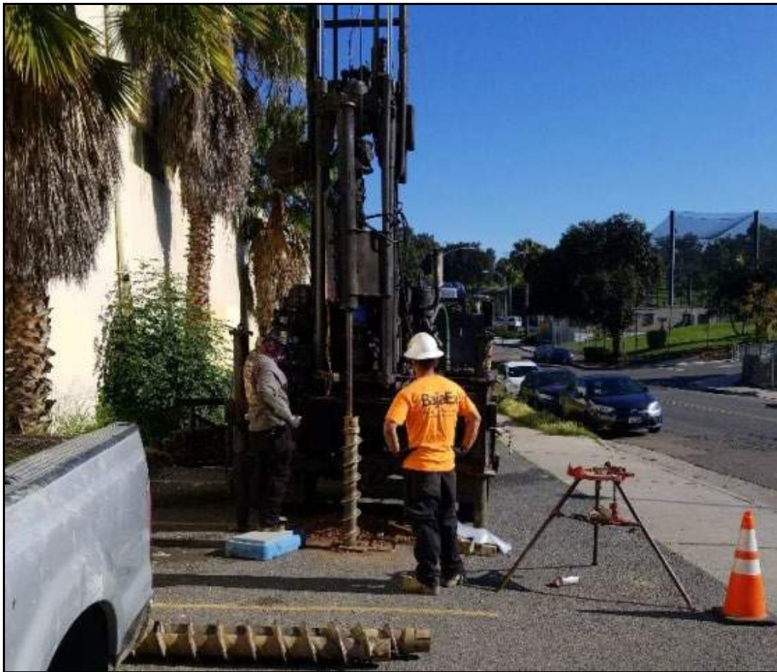
Figure 3-2. Drilling Operations, April 23, 2020
