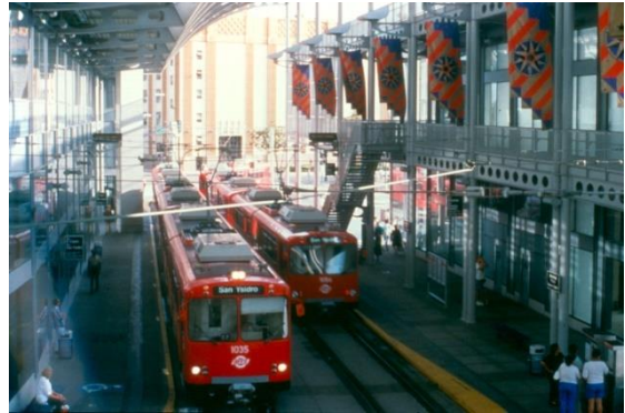
The American Plaza Trolley Station downtown provides an architecturally integrated, “front door” experience for transit patrons.
