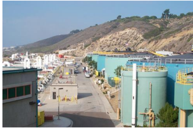
Point Loma Wastewater Treatment Plant
