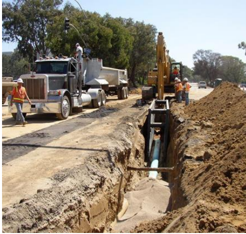
Trenching the municipal sewer system
