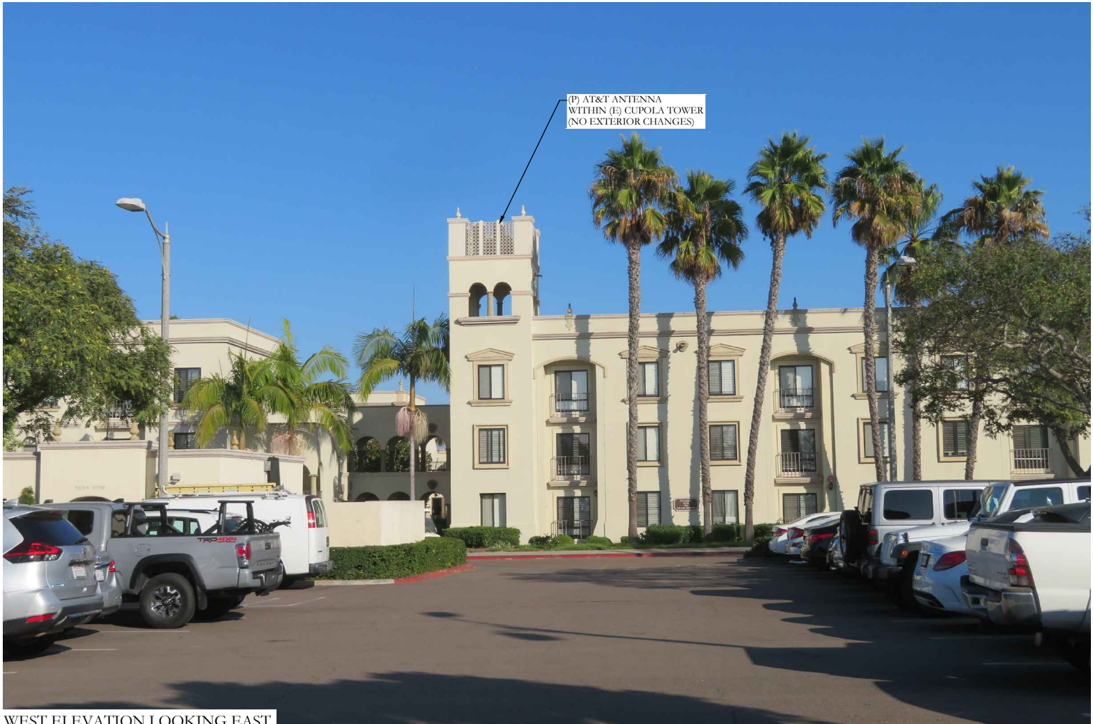
WEST ELEVATION LOOKING EAST
