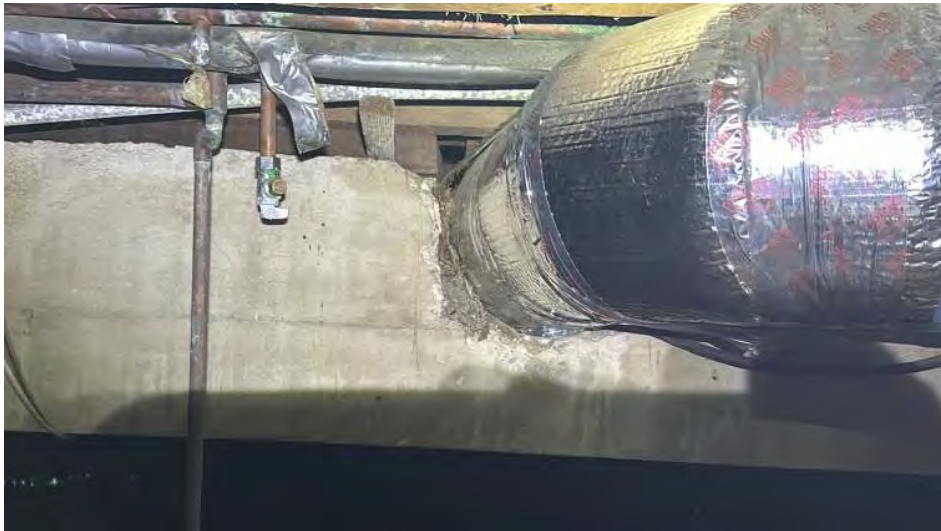
Figure C - Notch in foundation beam to accommodate ductwork.
