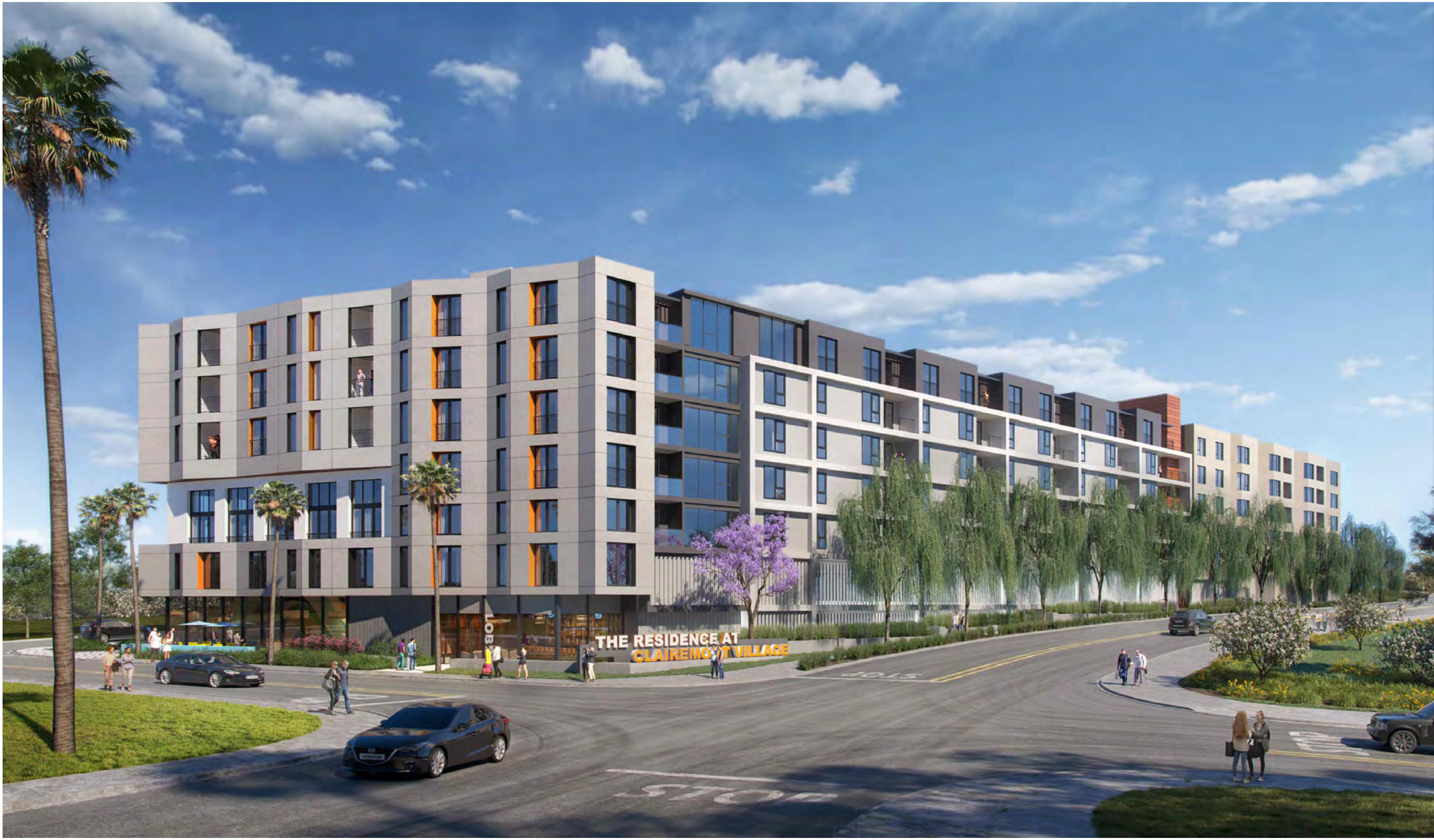
FROM COWLEY AND FIELD LOOKING NORTH 4
