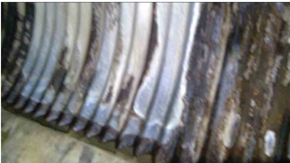
1873.00ft Infiltration Weeper from 3 o'clock to 5 o'clock, Finish
