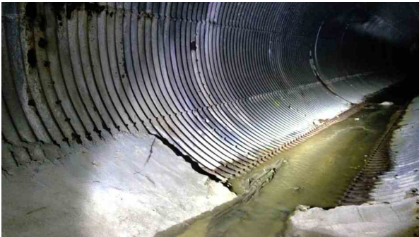
185.00ft Miscellaneous Material Change, Corrugated metal pipe / CMP
