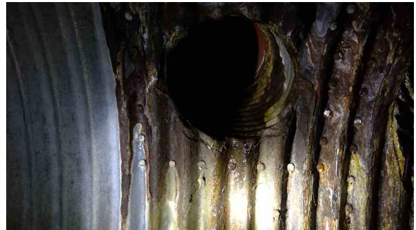
1732.00ft Tap Factory Made at 10 o'clock, dia/height: 24inch
