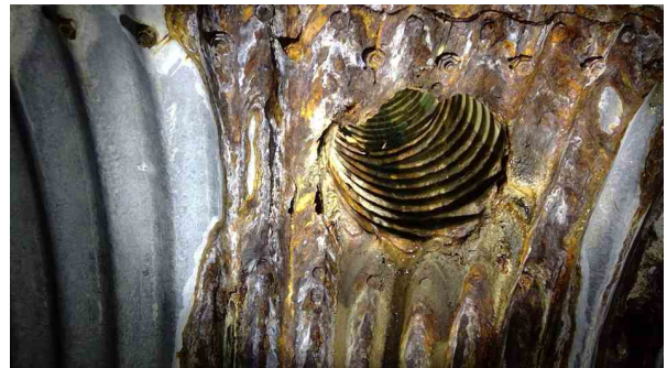
732.00ft Tap Factory Made at 10 o'clock, dia/height: 18inch
