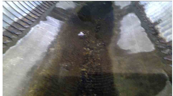
487.00ft Deposits Settled Fine, 10% of cross sectional area from 5 o'clock to 7 o'clock, Finish
