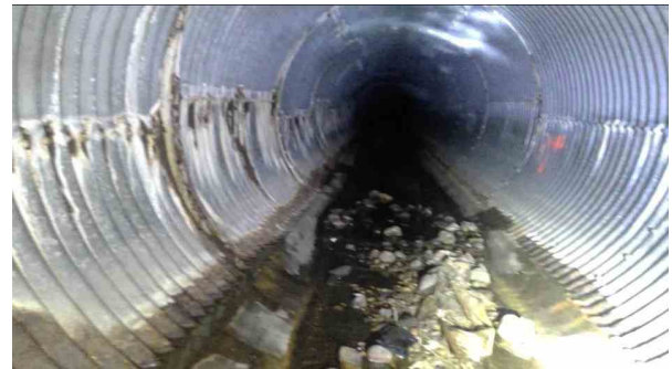
855.00ft Deformed Flexible Elliptical, change to: 10%, Finish
