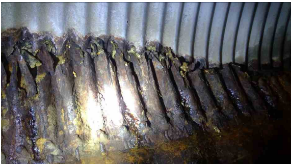
2586.00ft Surface Damage Corrosion from 7 o'clock to 9 o'clock, Start
