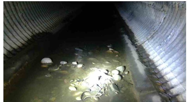
152.00ft Deposits Settled Other, 10% of cross sectional area from 4 o'clock to 8 o'clock / Debris
