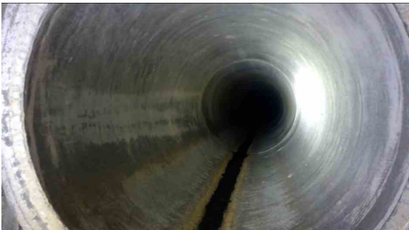
1198.00ft Tap Break-In Intruding at 9 o'clock, dia/height: 36inch, intruding: 12inch
