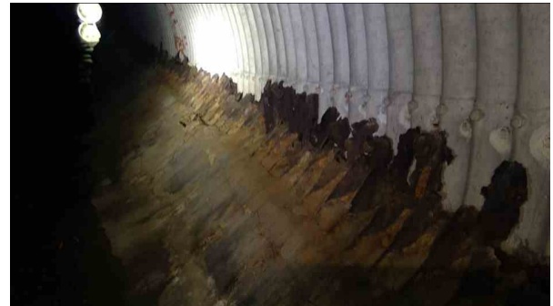
2586.00ft Surface Damage Corrosion from 3 o'clock to 5 o'clock, Start
