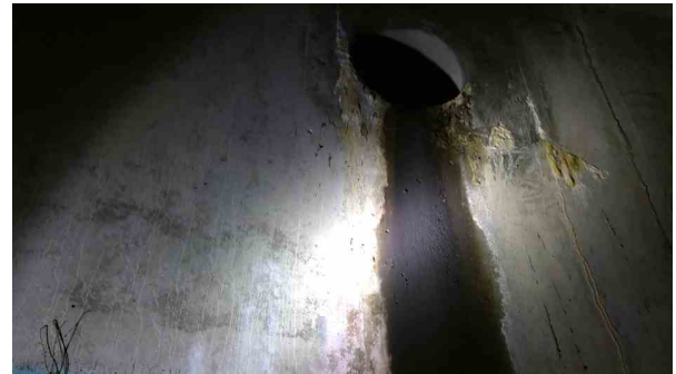
117.00ft Tap Factory Made at 11 o'clock, dia/height: 18inch
