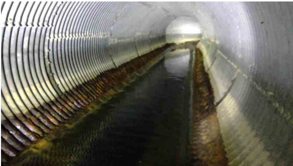
1305.00ft Obstruction Rocks, 15% of cross sectional area from 5 o'clock to 7 o'clock, Finish
