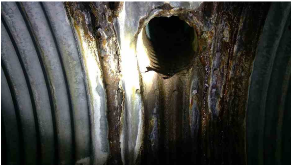
1904.00ft Tap Factory Made at 2 o'clock, dia/height: 18inch
