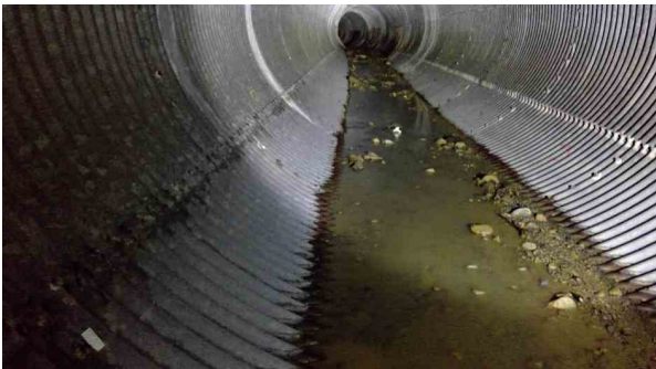
595.00ft Deposits Settled Other, 10% of cross sectional area from 5 o'clock to 7 o'clock, Start / debris
