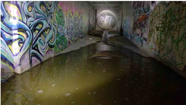
55.00ft Miscellaneous Shape or Size Change, dia/height: 99inch, width: 99inch / 14'X12' RCB
