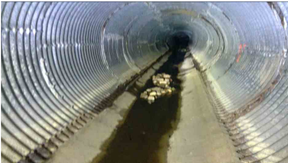
758.00ft Deformed Flexible Elliptical, change to: 10%, Start
