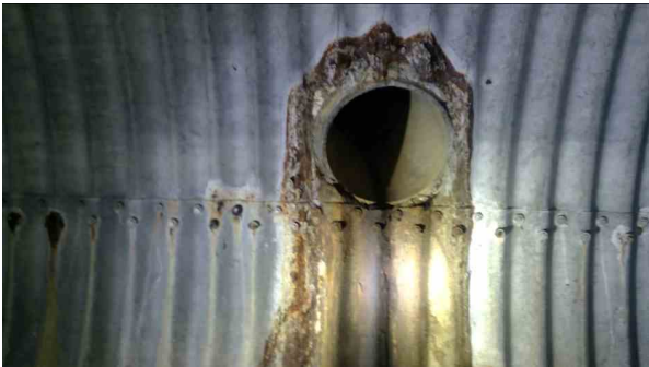
2580.00ft Tap Break-in/Hammer at 10 o'clock, dia/height: 18inch
