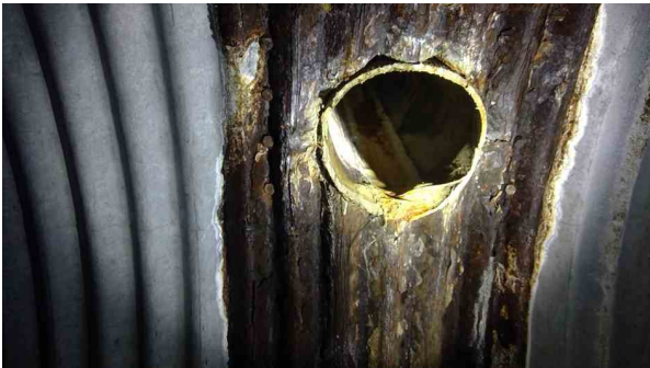
1930.00ft Tap Break-in/Hammer at 10 o'clock, dia/height: 18inch
