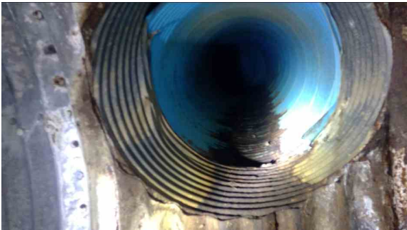
544.00ft Tap Break-in/Hammer at 11 o'clock, dia/height: 42inch
