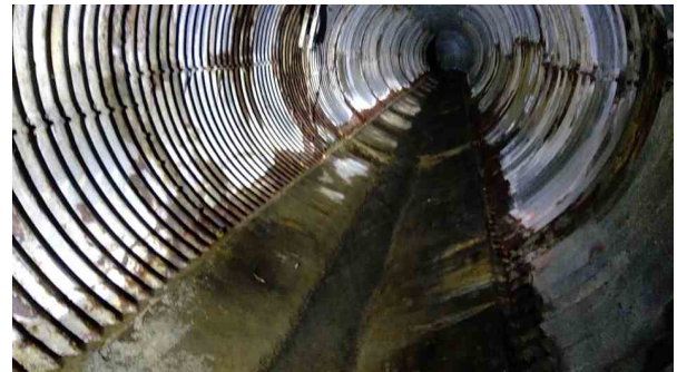
1025.00ft Miscellaneous Material Change, Corrugated metal pipe / cmp
