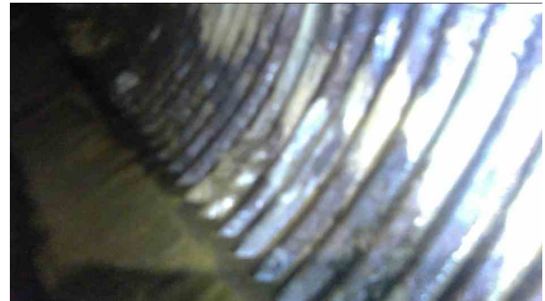
1850.00ft Infiltration Weeper from 3 o'clock to 5 o'clock, Start
