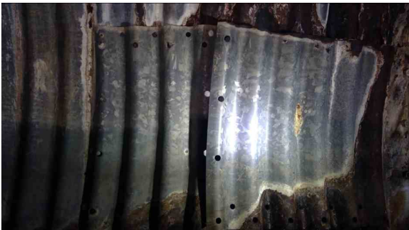
855.00ft Miscellaneous General Observation / Wall falling off
