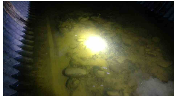
85.00ft Deposits Settled Other, 10% of cross sectional area from 5 o'clock to 7 o'clock / Debris
