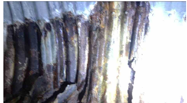
2035.00ft Deformed Flexible Bulging Inverse Curvature, change to: 5% from 2 o'clock to 4 o'clock
