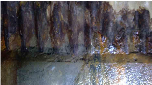
2762.00ft Infiltration Runnel from 4 o'clock to 5 o'clock
