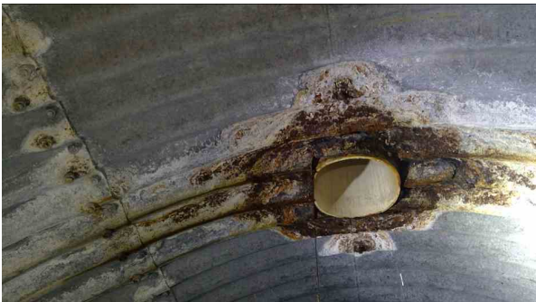
1050.00ft Tap Break-in/Hammer at 12 o'clock, dia/height: 15inch
