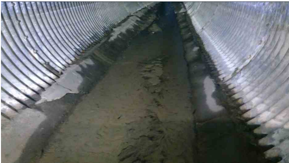
243.00ft Deposits Settled Fine, 10% of cross sectional area from 5 o'clock to 7 o'clock, Start
