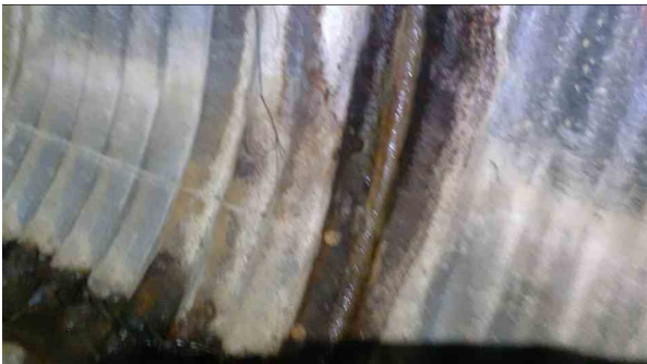
487.00ft Infiltration Weeper from 3 o'clock to 5 o'clock
