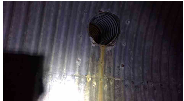
565.00ft Tap Factory Made at 10 o'clock, dia/height: 18inch
