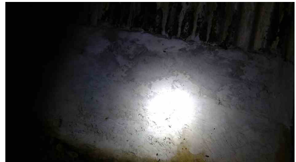
779.00ft Point Repair Patch from 7 o'clock to 9 o'clock / concrete
