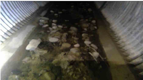
75.00ft Deposits Settled Other, 10% of cross sectional area from 4 o'clock to 8 o'clock / Debris
