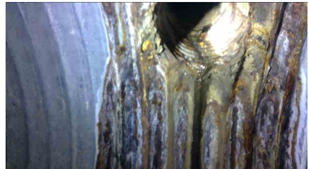
758.00ft Tap Factory Made at 11 o'clock, dia/height: 18inch
