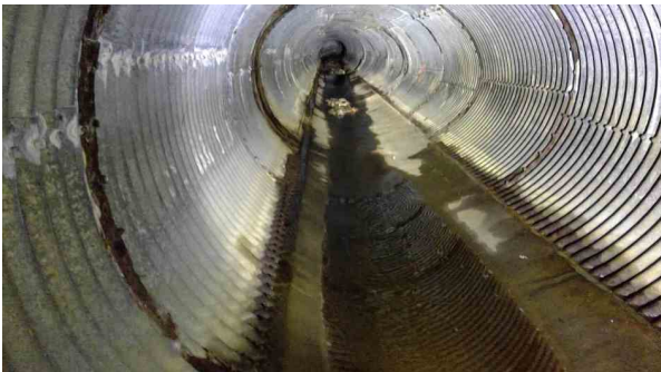
699.00ft Obstruction Rocks, 15% of cross sectional area from 5 o'clock to 7 o'clock, Start
