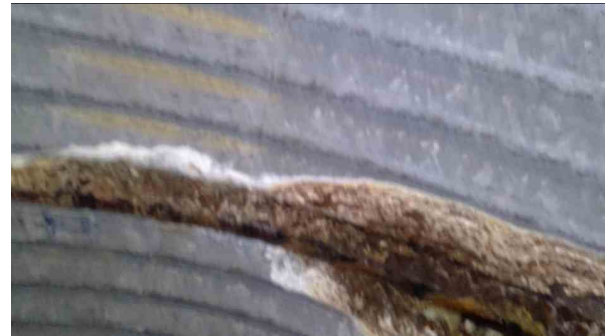
1007.00ft Infiltration Weeper from 8 o'clock to 4 o'clock, within 8 inch
