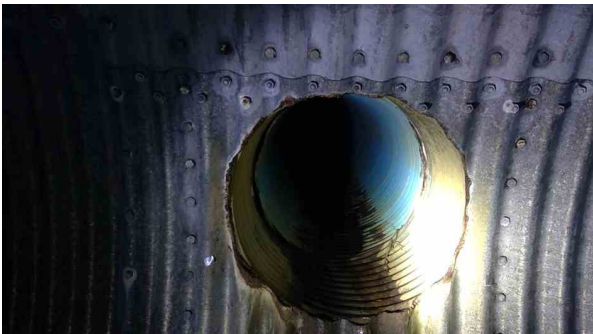
1404.00ft Tap Factory Made at 10 o'clock, dia/height: 36inch
