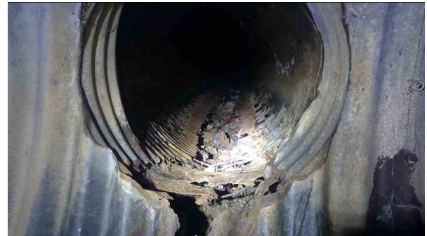
2762.00ft Tap Break-In Defective at 9 o'clock, dia/height: 36inch
