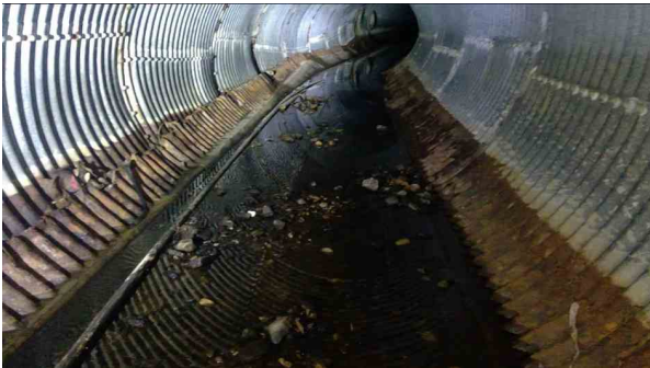
1083.00ft Deposits Settled Other, 15% of cross sectional area from 4 o'clock to 8 o'clock / Debris
