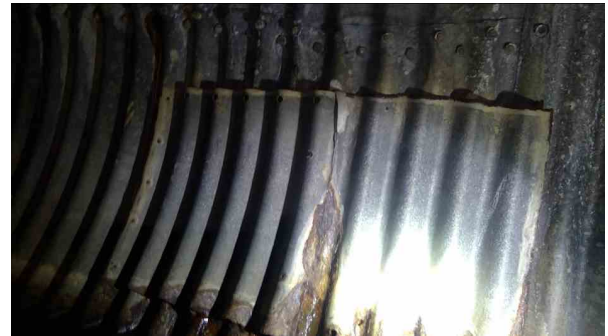
850.00ft Miscellaneous General Observation / Wall falling off
