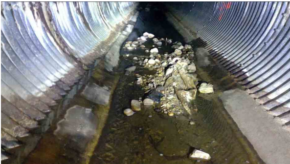
855.00ft Deposits Settled Other, 10% of cross sectional area from 4 o'clock to 8 o'clock / Debris
