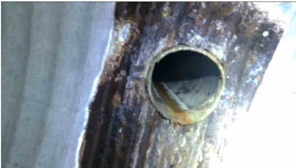
1946.00ft Tap Break-in/Hammer at 10 o'clock, dia/height: 18inch
