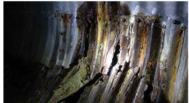
2023.00ft Fracture Multiple from 2 o'clock to 5 o'clock
