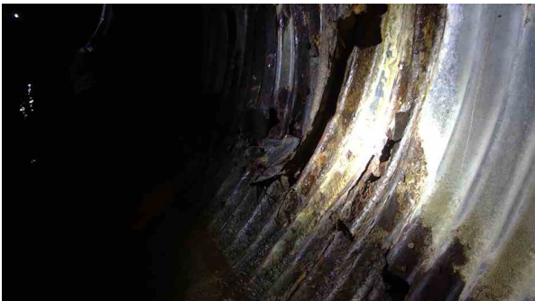
2011.00ft Fracture Multiple from 2 o'clock to 5 o'clock
