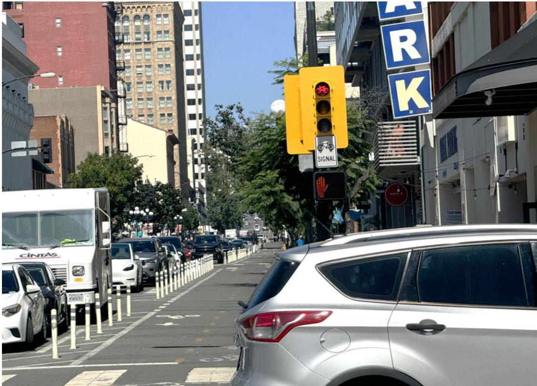
FIGURE 6-21 BICYCLE SIGNAL HEAD
