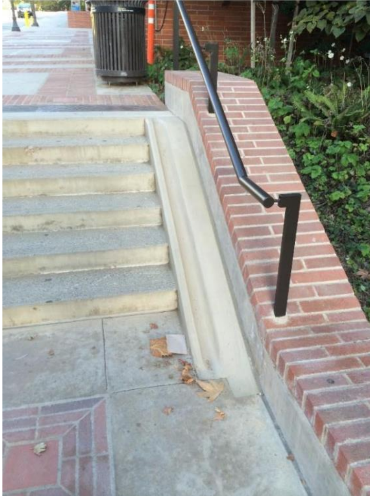
FIGURE 3-33 BICYCLE ACCESS CHANNEL
