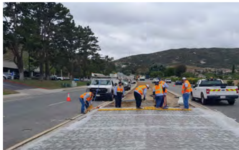
City crews constructing a center median.
