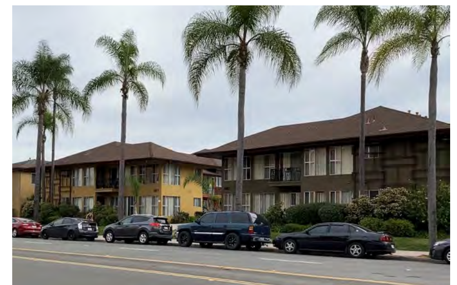
Multifamily homes give residents a variety of housing choices, including these garden apartments.
