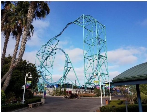
View of Electric Eel Coaster from within theme park
