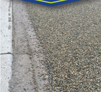
Completion of crushed rock layer prior to slurry seal application
