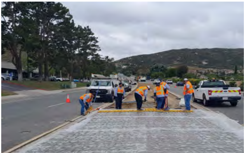
City crews constructing a center median.
