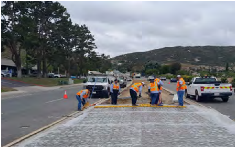
City crews constructing a center median.
