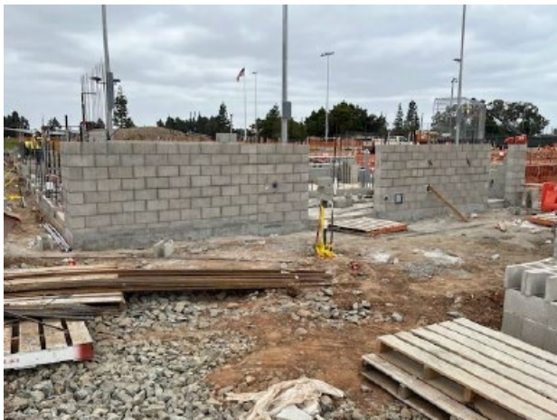
Ongoing installation of CMU at Equipment Building.
