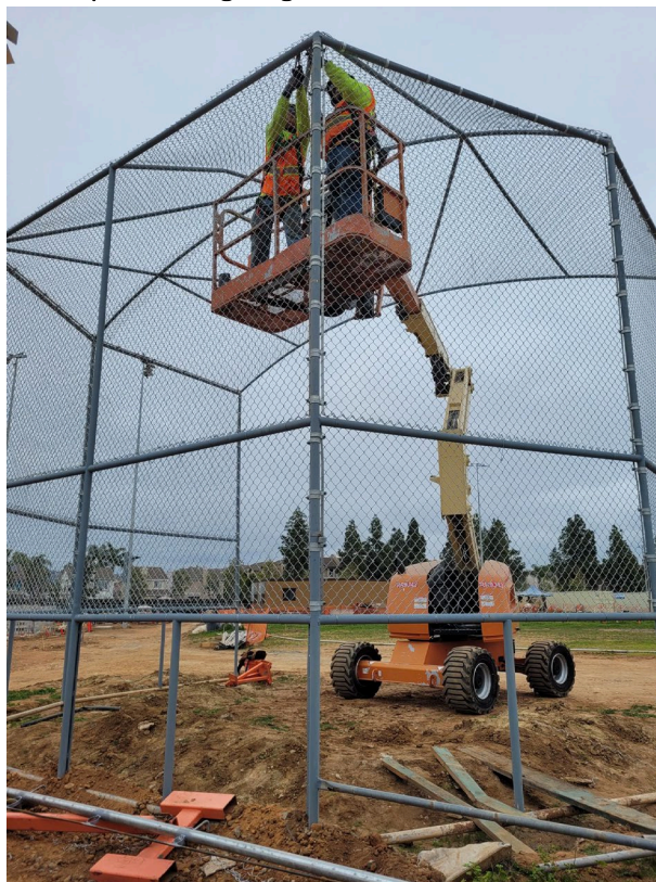
Installation of chain link at backstops are ongoing.
