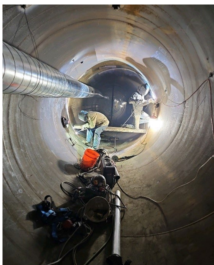
MCN I-805 Tunnel Casing Welding
