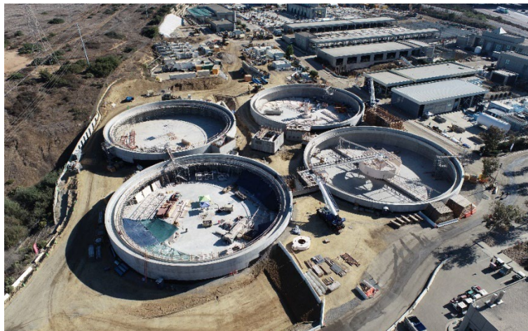
Pure Water NCWRP Secondary Clarifiers
