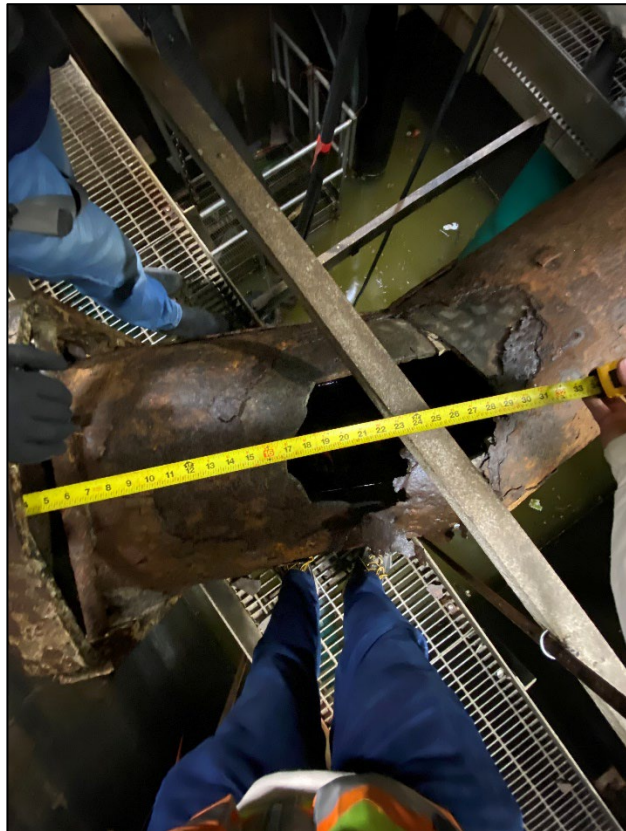
December 4, 2024 – Length of force main from pump flange to bend.
