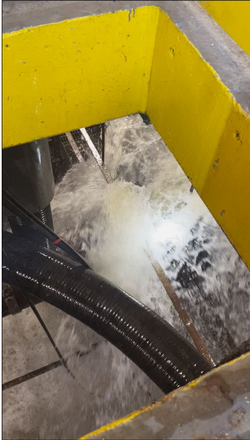
December 4, 2024 – Pipe failure during pump start up.
