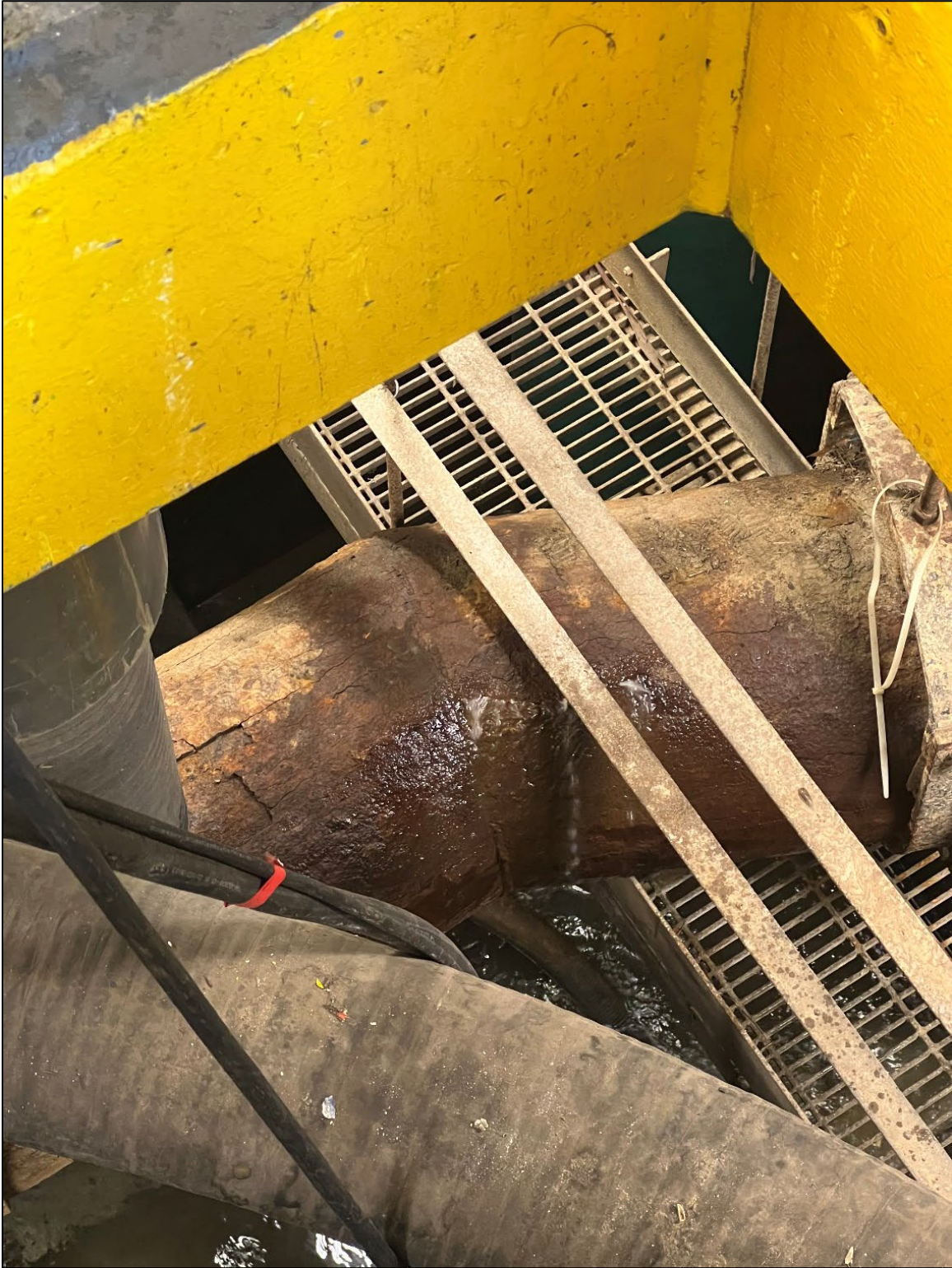
October 22, 2024 – Initial observation of stormwater leaking from 18-inch force main upstream of the 40-horsepower pump. Pump still operational.
