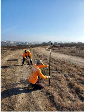
Photo 71. Contracted crew performing fence installation.
