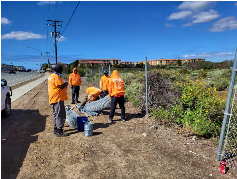
Photo 4. Contracted crew performing fence repair.
