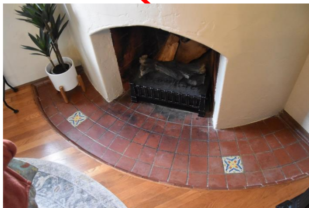
Detail of quarry tile fireplace hearth with D&G tiles
