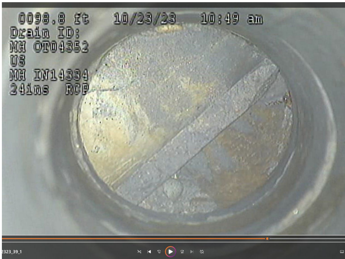
12-inch riser with debris per CCTV from October 23, 2023
