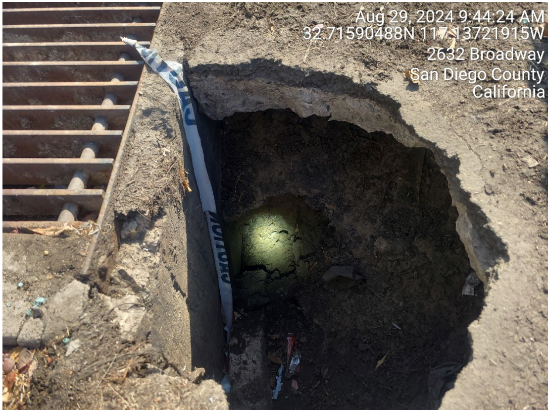
Sinkhole and undermined road in front of the catch basin
