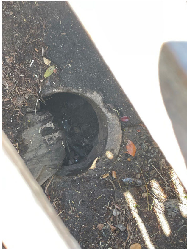
Broken 12-in riser within catch basin
