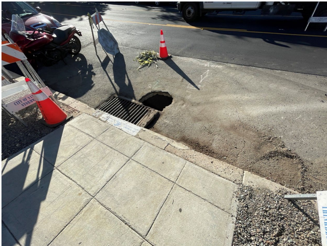
Sinkhole in front catch basin at 2650 Broadway St.
