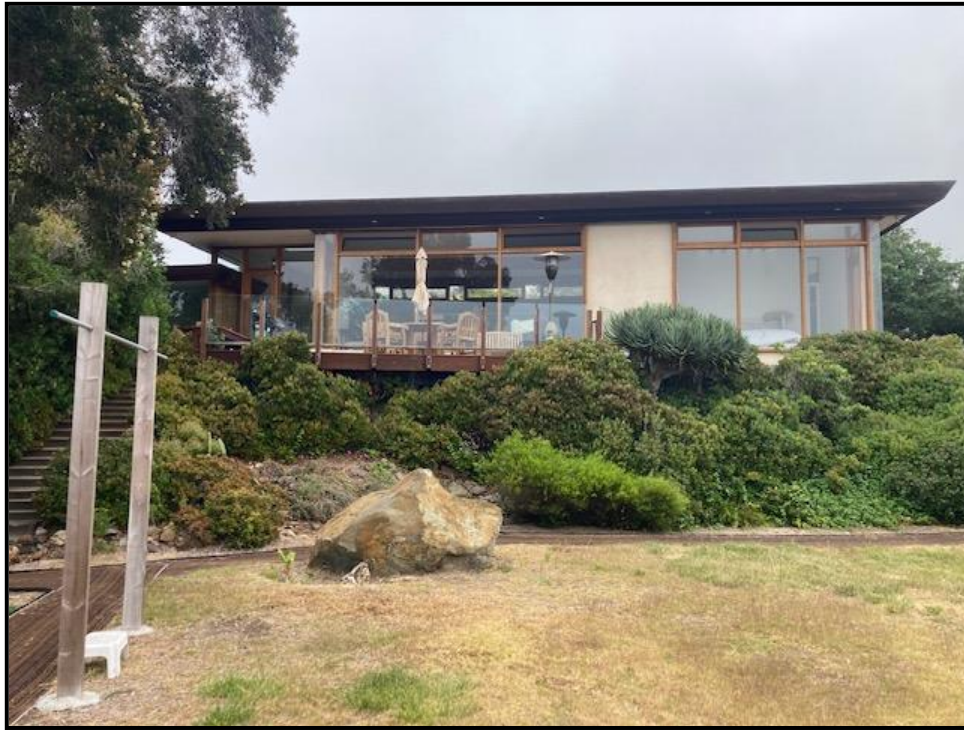
Plate 5: View toward the existing residence, facing south.
