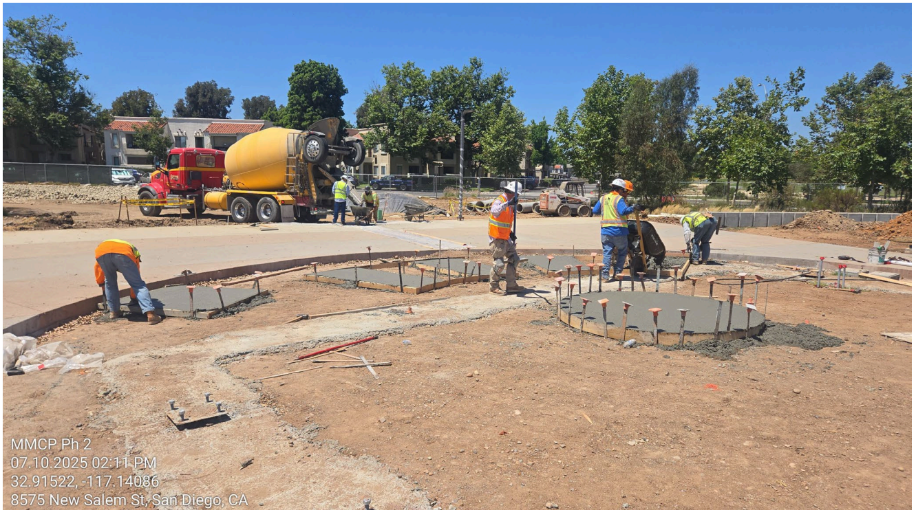
Mockup preparation for public art concrete
